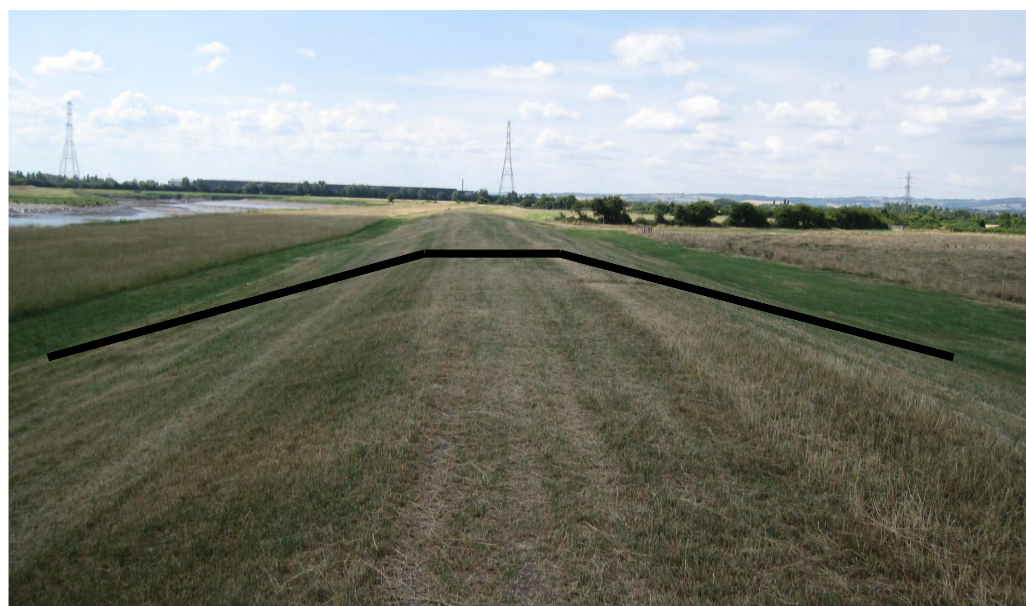
This image, of the flood banks at Cannington Bends, shows what the new and raised banks could look like. The lines indicate the profile of the bank.
