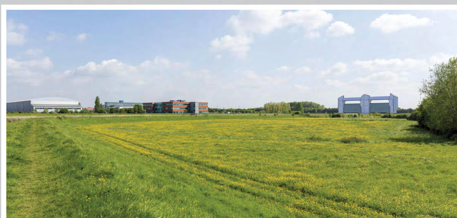
View south east from embankment footpath. Distance to barrier, 380 metres.
